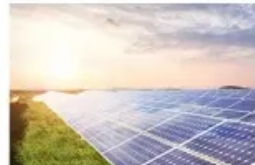
Energy Storage System
